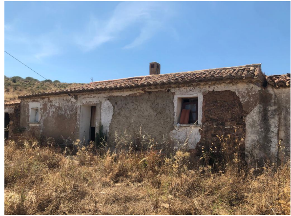
Fig. 1. Housing of rectangular floor plan in schist and rammed earth, plastered with lime, located in Bensafirim, Lagos.
