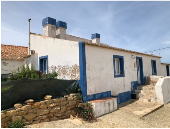
Fig. 3. Housing of rectangular floor plan in rammed earth, plastered with lime and sunrise oriented, located in Montinhos do Burgau, Lagos.
